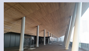
Exterior built using timber
