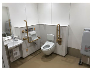
Accessibility in the restroom © Japan Sport Council
