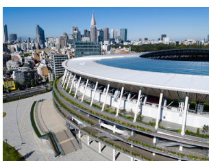
Grand eaves and skylight © Japan Sport Council
