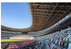
Integrated solar cells on the roof © Japan Sport Council
